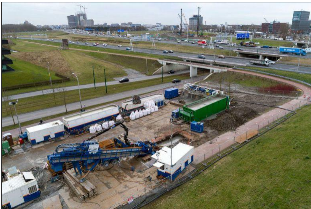
Figure 9-39 Example of Construction Site Layout for Horizontal Directional Drilling
