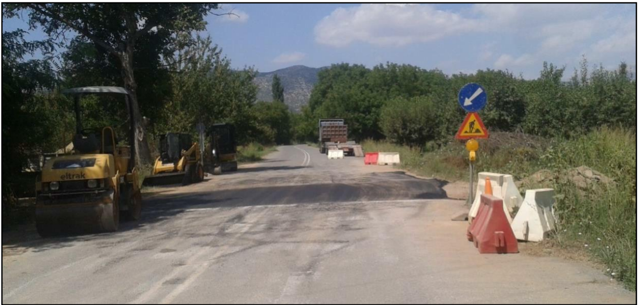
Figure 9-40 Example of Restoring Road Surface and Traffic immediately after Open cut
