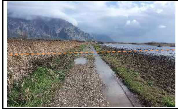
Source: Project FEED, 30-10-2020. Orange line roughly indicates pipeline route.
